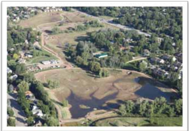
The Canal Importation Ponds and Outfall (CIPO) Drainage Improvement Project will reduce flooding risk, improve water quality, and restore and enhance the Red Fox Meadows Natural Area.
