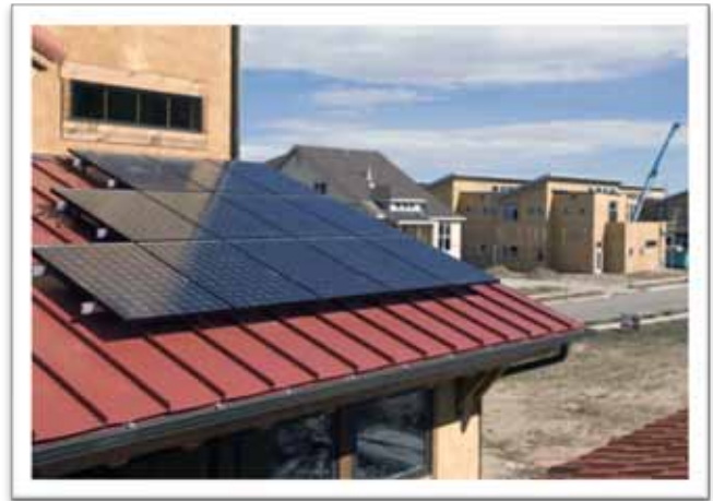
Incorporation of renewable energy sources into new development is encouraged, like the inclusion of solar panels on the roof of this new home.
