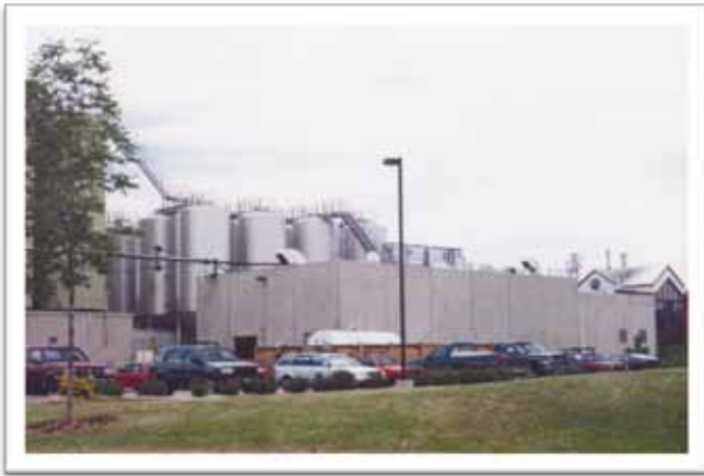
A typical Industrial District located in northern Fort Collins.
