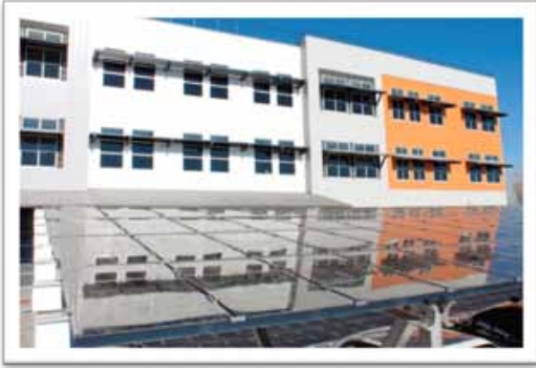
The recently completed Innosphere (formerly Rocky Mountain Innovation Initiative) building will incubate, support and accelerate the success of innovation-based startup companies in Northern Colorado.
