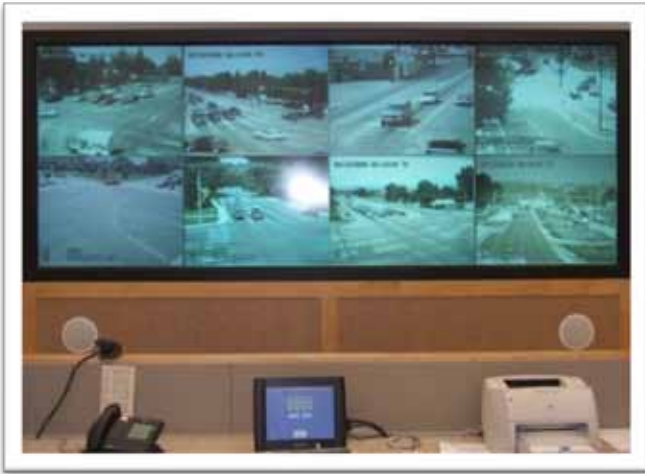
The Advanced Traffic Management Center helps monitor and manage the City's transportation system.
