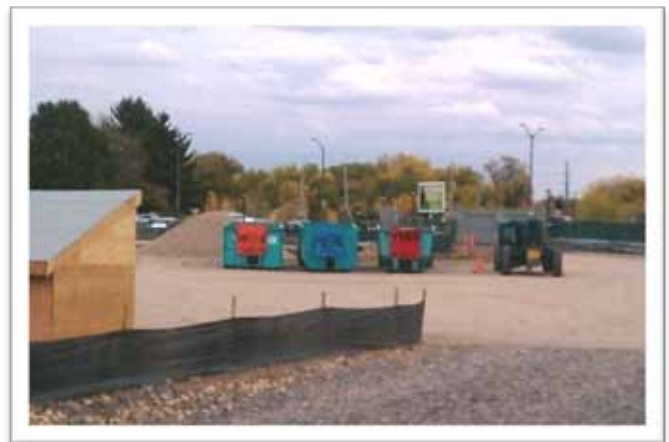
Sorting and recycling of construction-related materials can significantly reduce the amount of waste sent to landfills.
