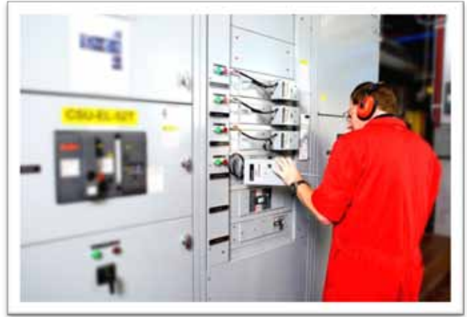
Modernization of the electric grid can enable flexibility and automation of the electric grid, provide real-time feedback to users, and reduce energy use.
