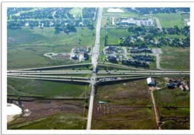
Future improvements to the Interstate 25 and Highway 392 interchange are a result of regional cooperation between the City of Fort Collins, Town of Windsor, and Colorado Department of Transportation.
